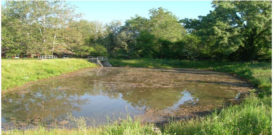
Water treatment residual storage lagoons were near capacity prior to commencement of the project.
