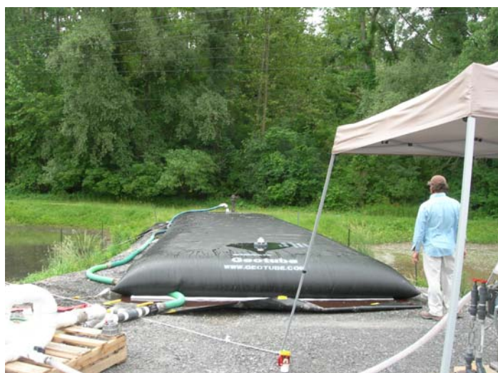
The Geotube® container after filling commenced.
