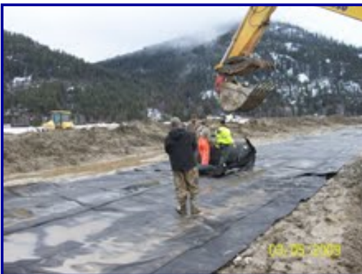
(Left) Placing Geotube® unit on scour apron.
