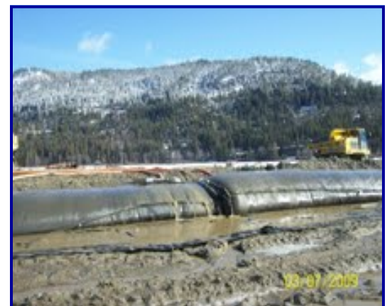
(Right) Filled Geotube® units.
