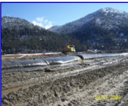
(Left) Filling Geotube® units using flatend technology.
