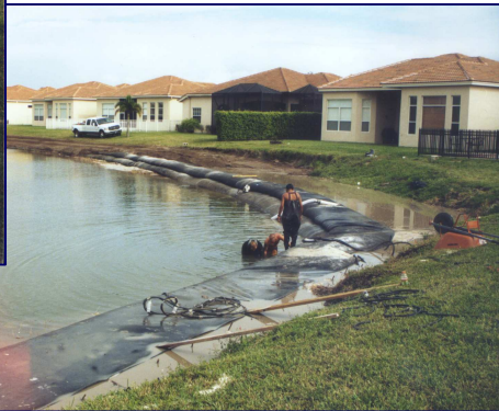
Geotube® LES™ being installed
