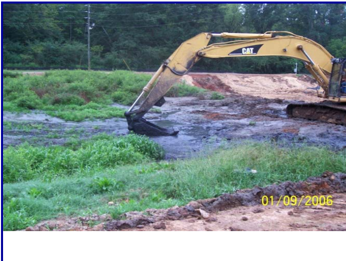
Mechanical excavation of vegetation and other debris from a 1-MG biosolids storage lagoon prior to hydraulic dredging to Geotubes® containers for further processing (i.e., dewatering and consolidation).
