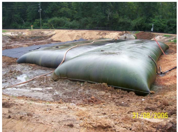
The south storage lagoon was used for Geotube® containers after initial excavation of biosolids into the north lagoon.
