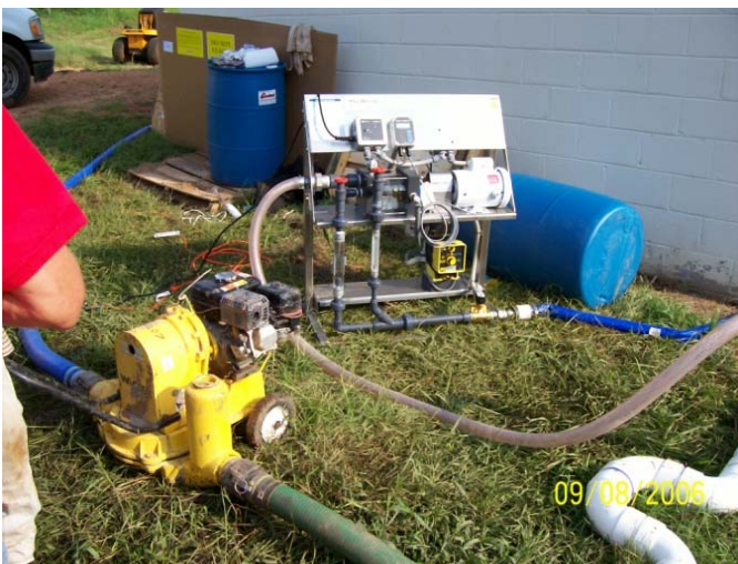
Injection of polymer with WaterSolve's WSLP-2400 make down unit.
