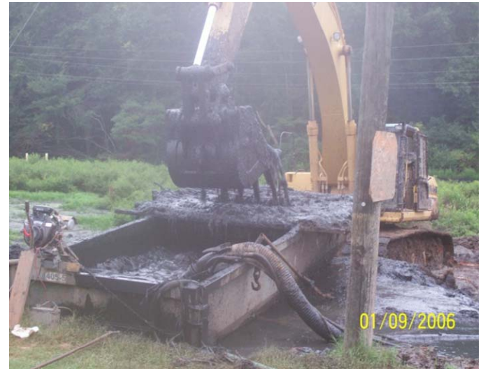
Mechanical excavation of vegetation and other debris from a 1-MG biosolids storage lagoon prior to hydraulic dredging to Geotubes® containers for further processing (i.e., dewatering and consolidation).
