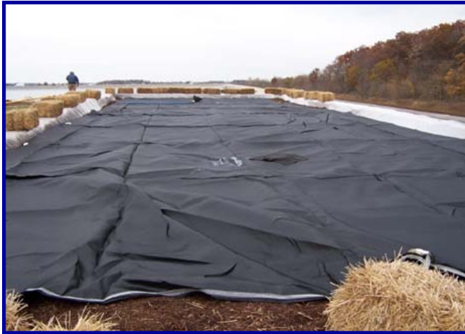
One hundred ft. 60-ft circumference Geotube®
