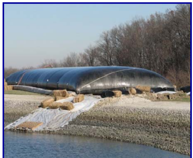
Geotube filled to maximum height 7 ft.
