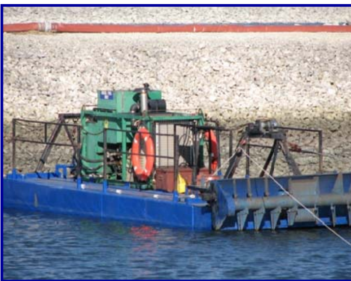
This cable dredge transferred the residuals from the lagoon to the Geotube® container.
