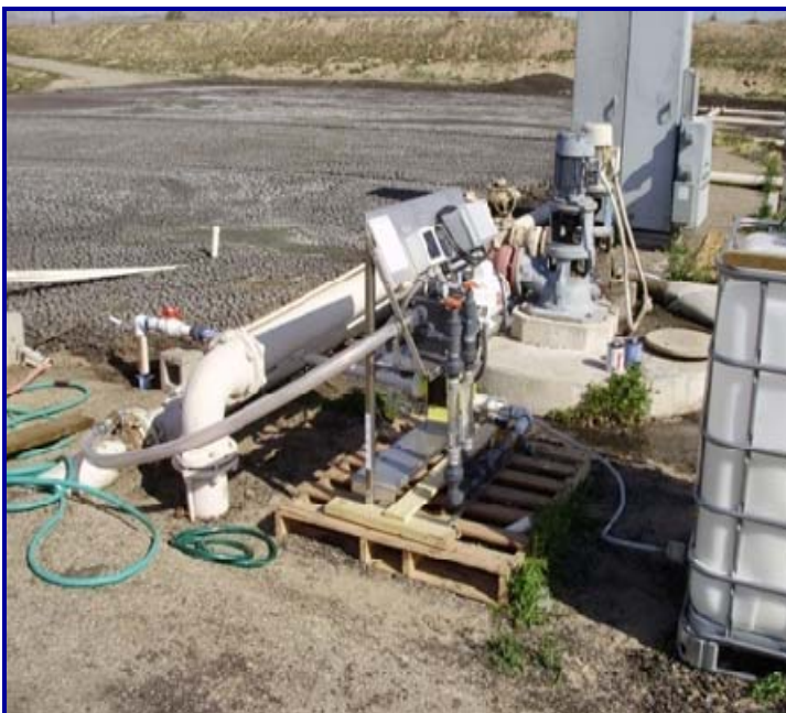
The WSLP-2400 polymer make-down unit is delivering 2.5-gph of polymer to the 300-gph stream of biosolids.
