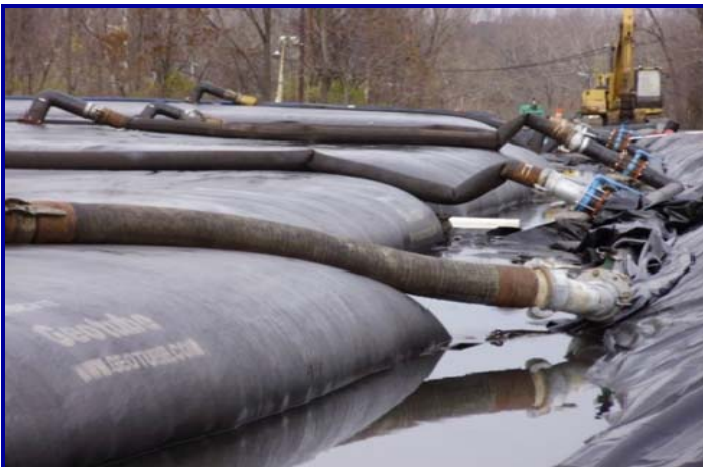
Geotube® containers were filled .
