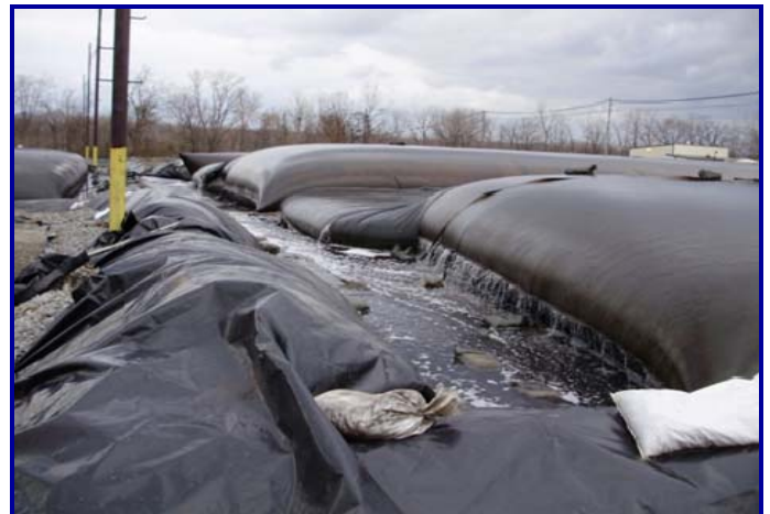
Supernatant from the Geotube® containers was diverted and
