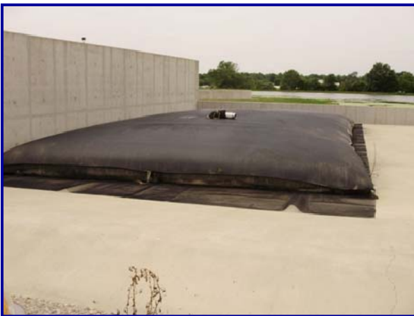
The Geotube® lies in the containment area atop of the drainage netting which allows the water to exit from the bottom of the tube.
