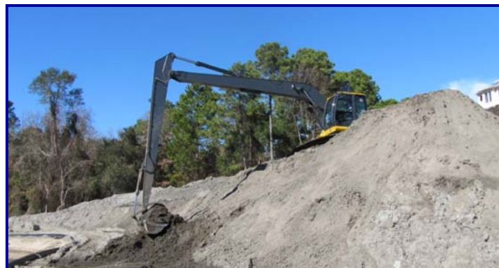
The long reach excavator dipped sand and mud out of the lagoon to maintain settling space for the water. It was then hauled and stockpiled for distribution at the end of the project.
