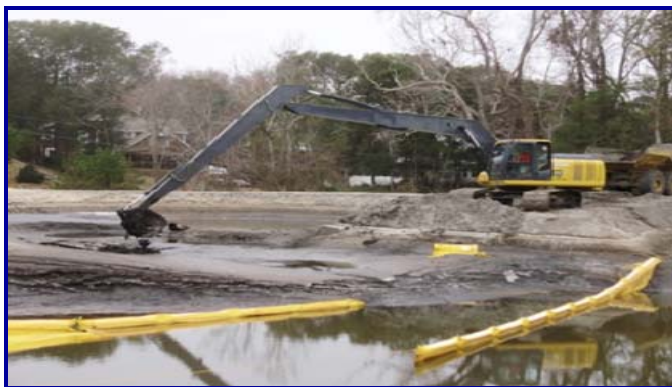
The long reach excavator dipped sand and mud out of the lagoon to maintain settling space for the water. It was then hauled and stockpiled for distribution at the end of the project.
