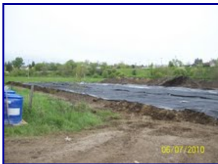
Geotube® container laid out on top of liner and GFF mat.
