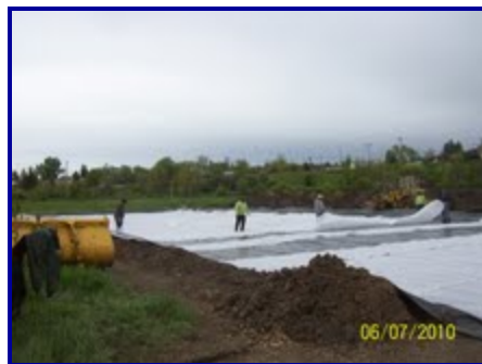
Laying out GFF mat on top of liner in containment area.
