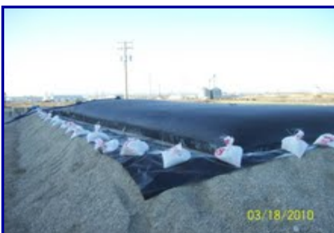
Geotube® container filled and dewatering.
