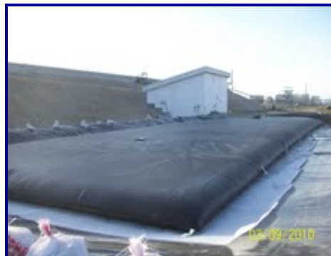
Dewatering of Geotube® container.
