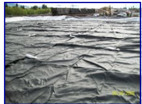
Containment area preparation.
