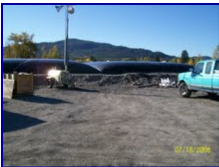
Containment area with Geotube® containers filled.
