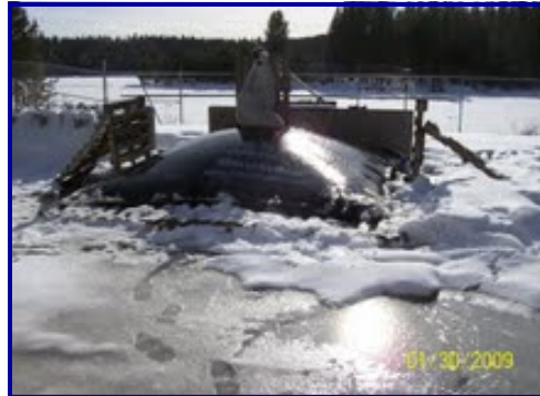
Winter operations filling and dewatering Geotube® unit.
