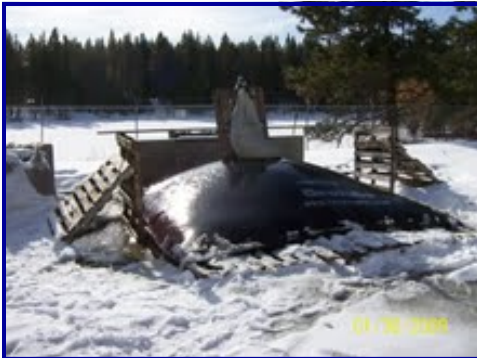
Winter operations filling and dewatering Geotube® unit.
