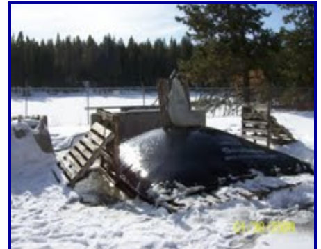
Winter operations filling and dewatering Geotube® unit.
