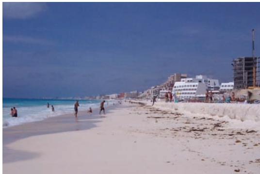
The same view, after Geotube® repair and restoration technology. The beach is coming back.
