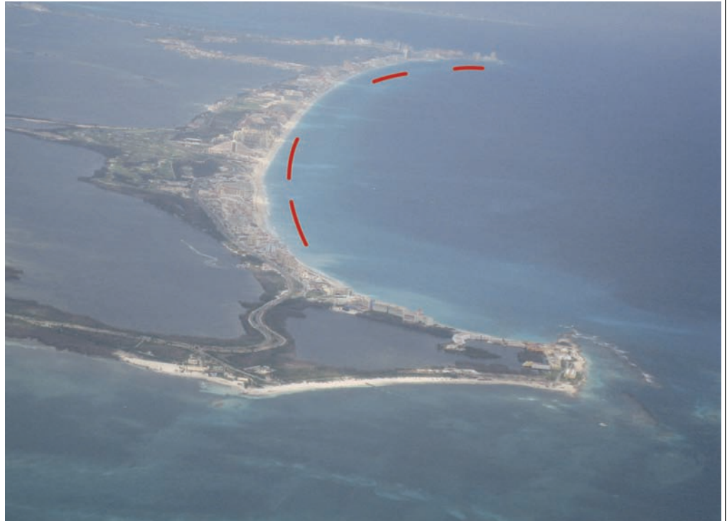
The red lines indicate the placement of a 4-section breakwater off Cancun's shoreline built with Geotube® containers. By changing wave patterns, this will help replenish the hurricane-damaged beach and protect ocean-front resort property from future erosion.
