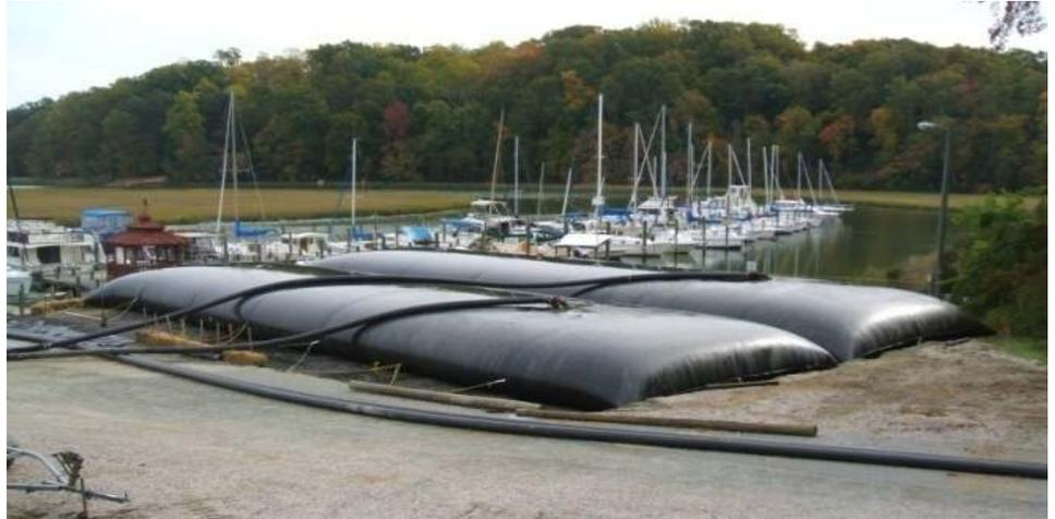
The filling and consolidation phase of the Geotube® containers took place over a two-week period.
