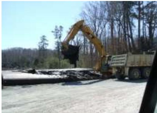
This project was started in November '07 and dredging was completed within two weeks. The Geotube® units were pumped to the maximum allowable height of 7.5', allowed to dewater and consolidate and then pumped to the maximum 7.5' height again. The material was left in the Geotube® containers through the winter. The dredged sediments continued to desiccate over the winter and were successfully transported off-site.
