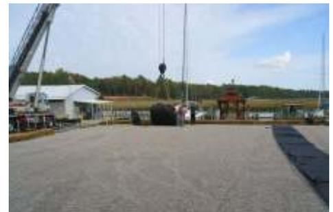
The Marina parking lot was used to construct a dewatering cell. The site was graded flat and #57 stone was placed for drainage under the Geotube® units. 60' circumference tubes are rolled onto steel cores for shipping and deployment on the site.
