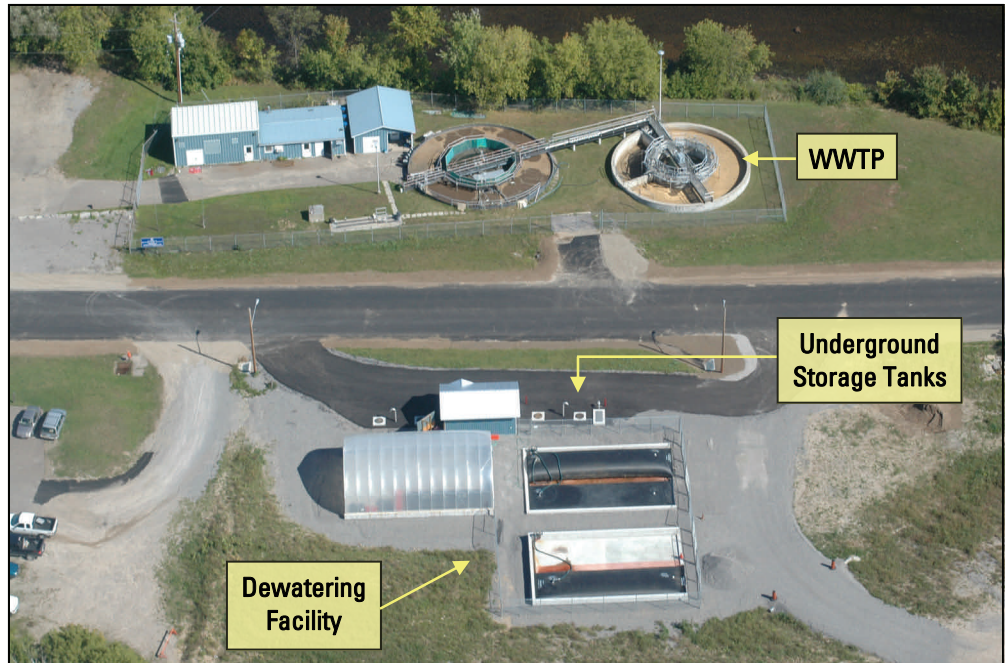
This aerial image shows the Biosolids / Septage Dewatering Facility directly across from Eganville's existing wastewater treatment plant. Underground septage storage tanks were incorporated at the site, allowing pumper trucks to easily offload septage materials. Geotube® dewatering cells are shown at bottom of photo.
