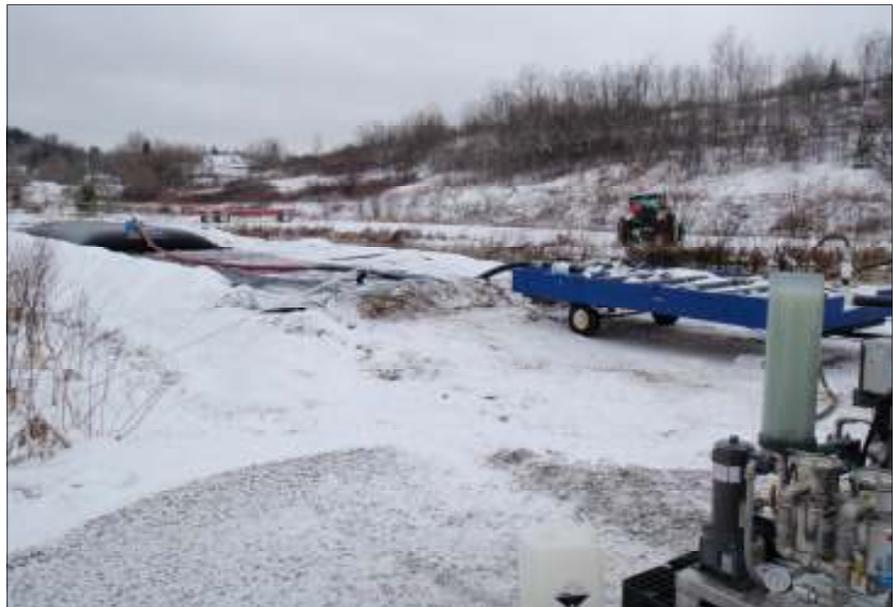
*Geotube® unit is being filled with sludge from the forebay in subzero temperatures, allowing a clear effluent to filter through the material of the bag and back into the forebay.*
