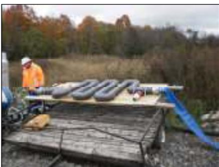
Sludge is injected with a polymer and transferred through the PVC mixing system prior to being dewatered.
