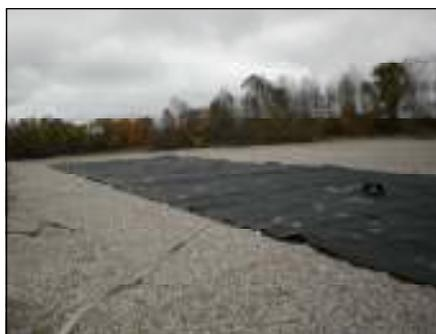
Lay down area constructed using a geo-membrane liner covered in crushed stone.
