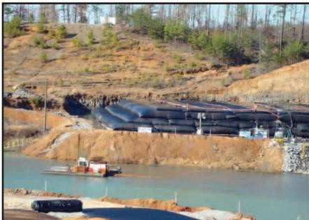
A dredge pumped slurry waste from the lagoon to the Geotube® containers.
