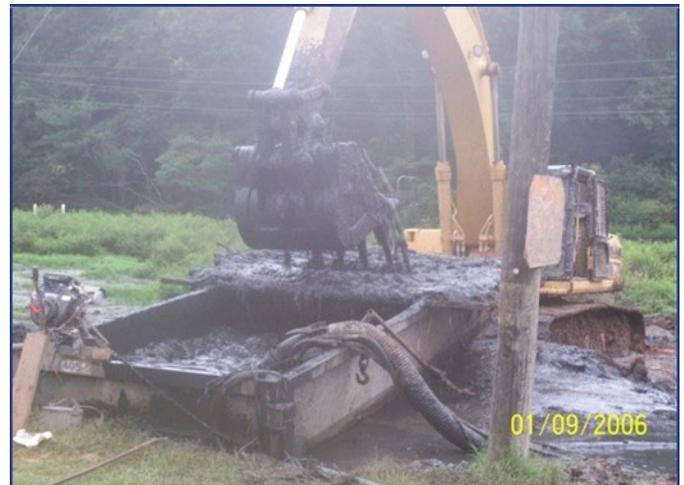
Mechanical excavation of vegetation and other debris from a 1-MG biosolids storage lagoon prior to hydraulic dredging to Geotubes® containers for further processing (i.e., dewatering and consolidation).
