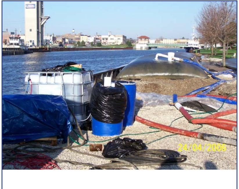
The 30'x90' and 30'x50' Geotube® containers were installed to contain and dewater 8 months of drilling residuals with less than 40 mg/L TSS in the filtrate. A key element in the release of water from drilling residuals is proper polymer mixing and injection to provide good chemical conditioning.
