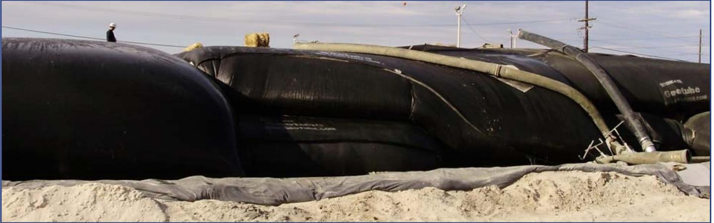
Geotube® containers were filled to the maximum height of 7.5-ft.
