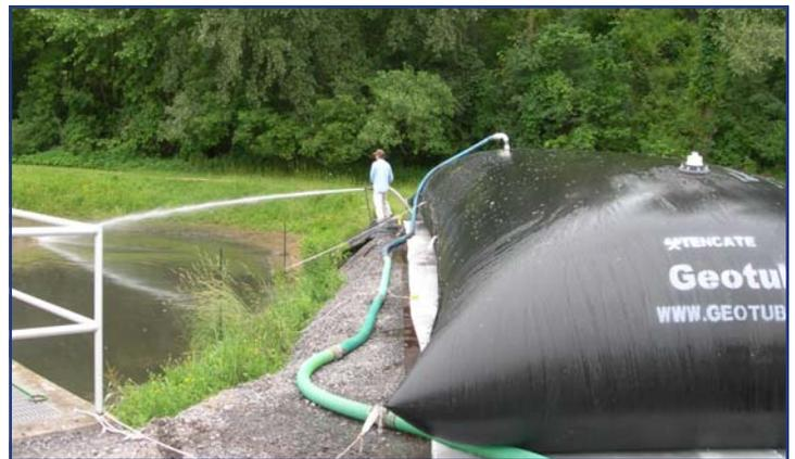
The lagoon residuals were homogenized by high-pressure spraying. The Geotube® container is being filled and is dewatering properly.
