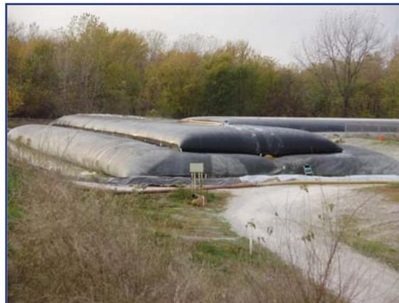
The Geotube® container is stacked to make the most of the space available at this site. .
