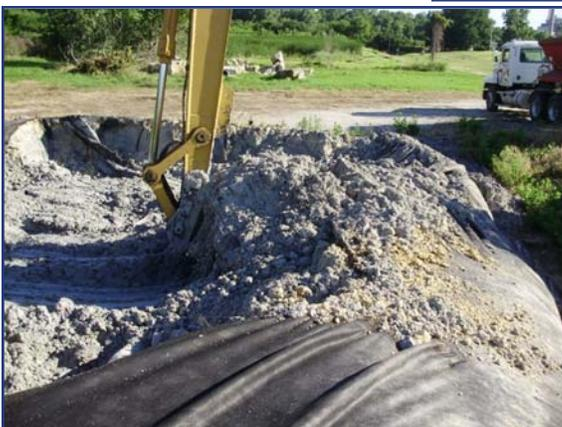
The residual in the Geotube® containers is being hauled away with dry wt solids ranging from 25 to 33%.
