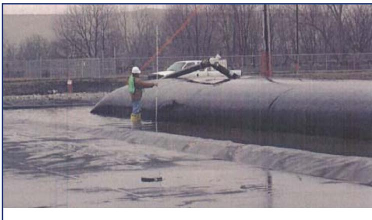
Geotubes® containers were periodically measured for fill height .
