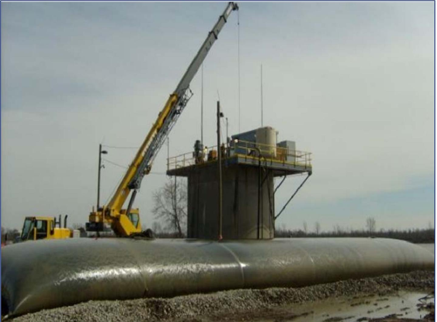
The Geotube® container after it is nearly full. The river intake well structure adjacent to the Ohio river shown in the background.
