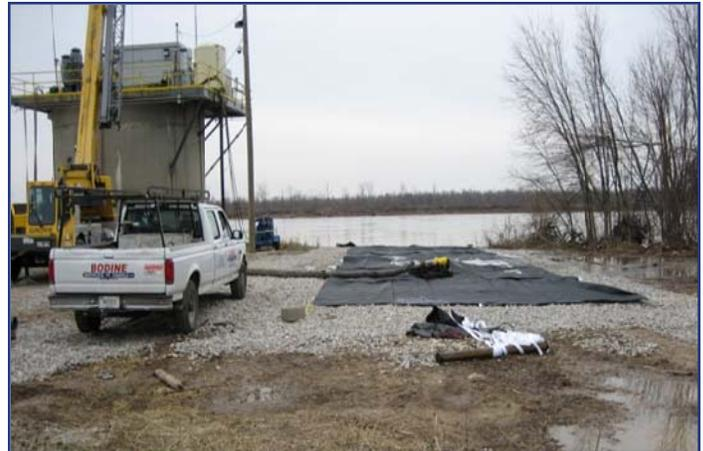
The water intake well shown at the left portion of the photograph was cleaned out. The sediment was dewatered in the Geotube® container shown. A stone pad was prepared for the lay-down area. The river is shown in the background.
