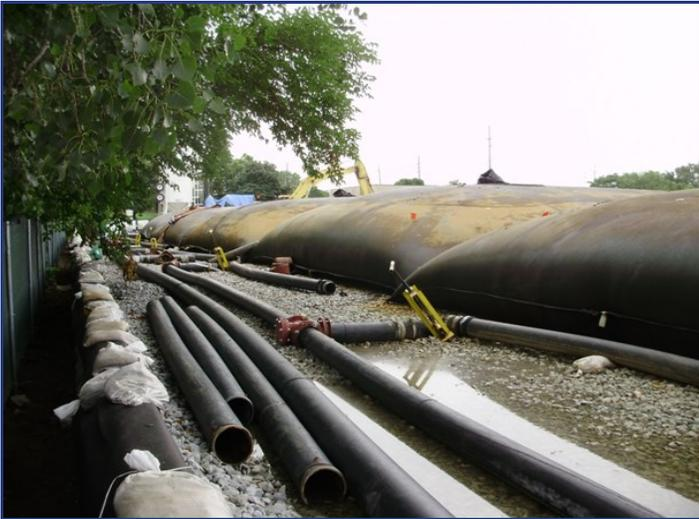
These Geotube® containers are full and will dry for several days before the material is handled.
