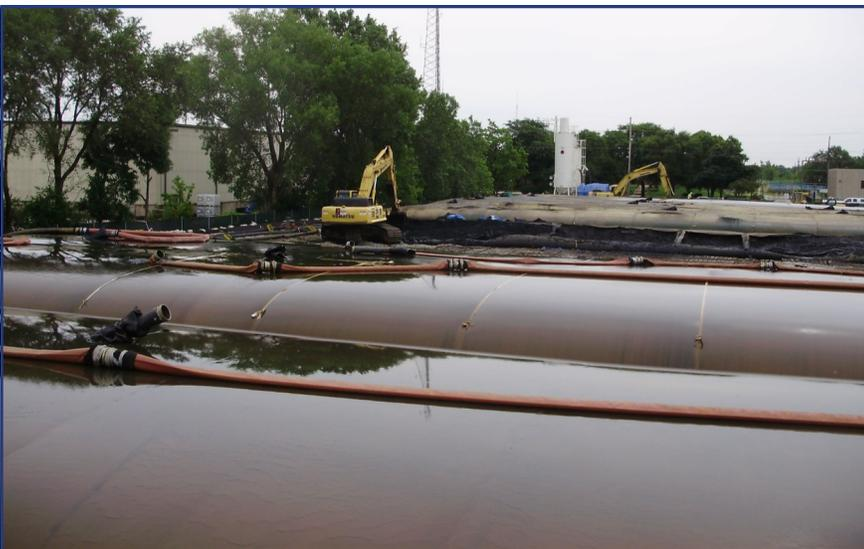
This containment area has capacity for eleven 75' circumference by 200' long Geotube® containers. As the material dries, and the bags are excavated and removed, new Geotube® containers are placed and filled. This system allows for continuous dredging operations.
