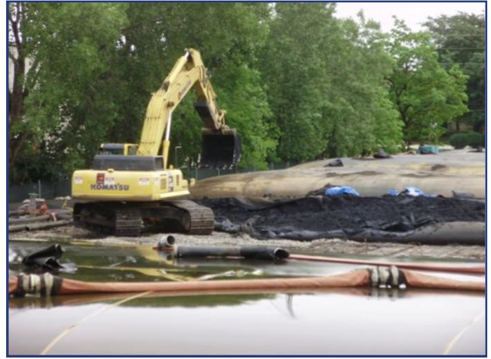
After being allowed to dewater, the bags and material were loaded and hauled away to a landfill for permanent disposal.
