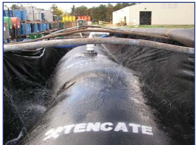
The Geotube® container filled to capacity and dewatering with tiny sprayers exiting the tube.
