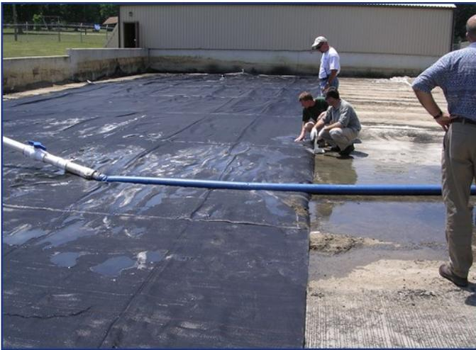
A 60' x 100' Geotube® container was installed to contain and dewater 12-18 months of biosolids (approximately 700,000 gallons).
