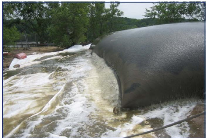
Water (filtrate) released from the Geotube® containers.
