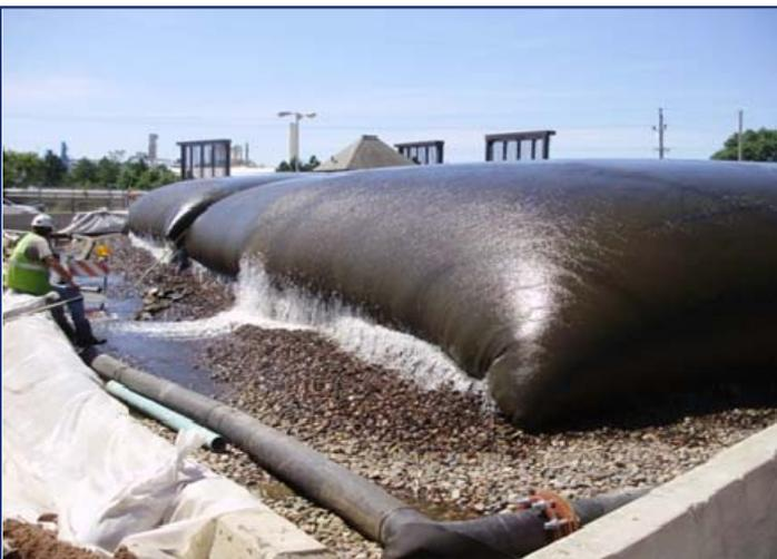
The Geotube containers were placed on a prepared pad of crushed stone. They are shown above in operation releasing clear filtrate.
