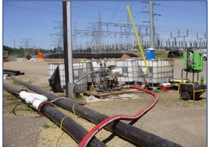
A polymer make-down unit is plumbed to the mixing manifold in the 8” supply line on its way to the Geotube® containers delivering 12 gallons of Solve 216B emulsion polymer per hour.
