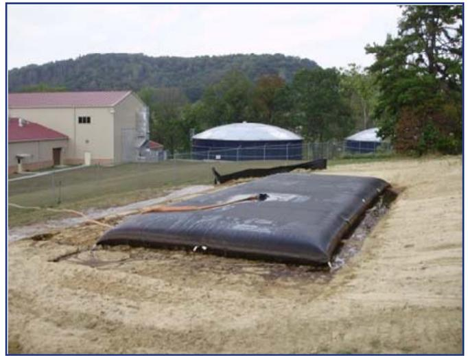
The Geotube® container lies on a level bed of sand for good drainage.
