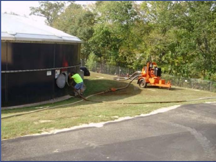
This backwash settling basin in Ohio is being agitated and pumped to a Geotube® container for dewatering and subsequent hauling to a landfill.
