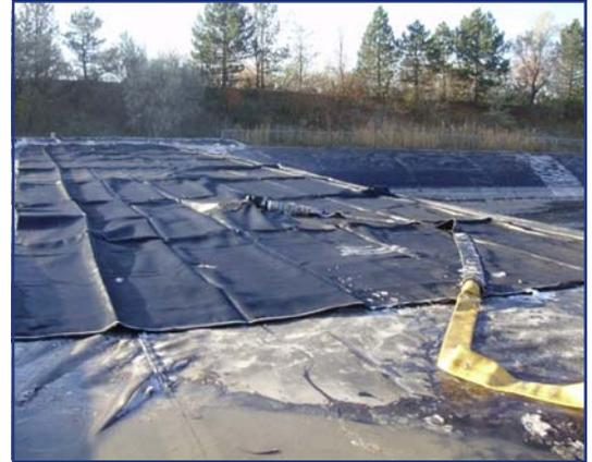
This Geotube® container was placed on the containment pad at the end of the holding pond and the filtrate drained back into the pond.
