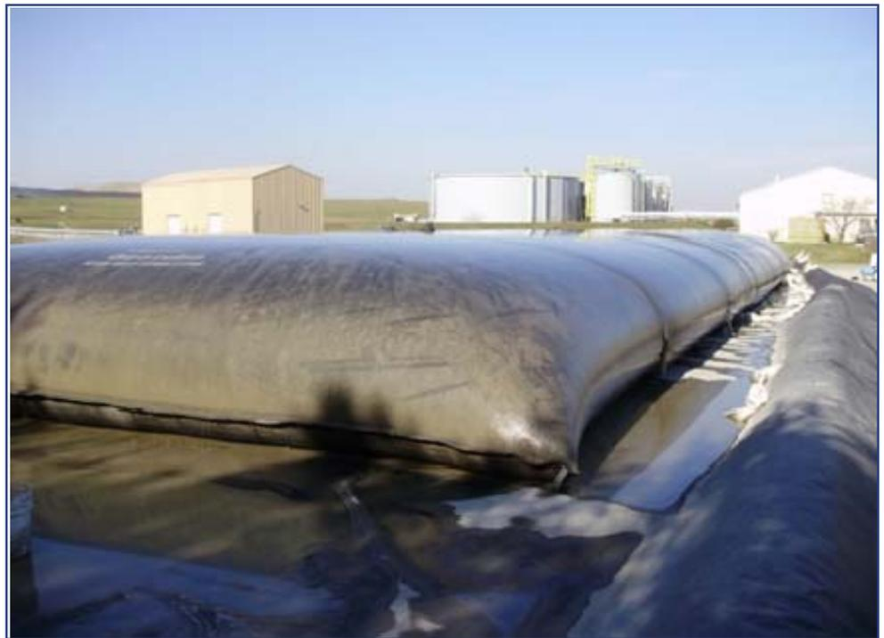
The Geotube® container is continuing to dewater. It was filled in November and will be excavated in the upcoming summer.
