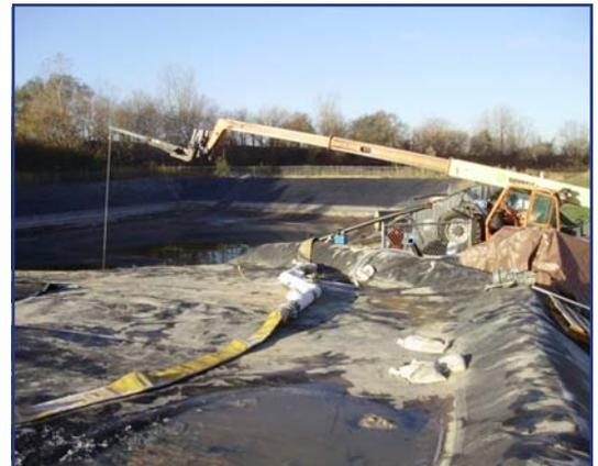
The telescoping forklift is holding the hydraulic pump in the settling pond and the 6" hose coming from that pump is connected to the white mixing manifold in which the polymer is injected.
