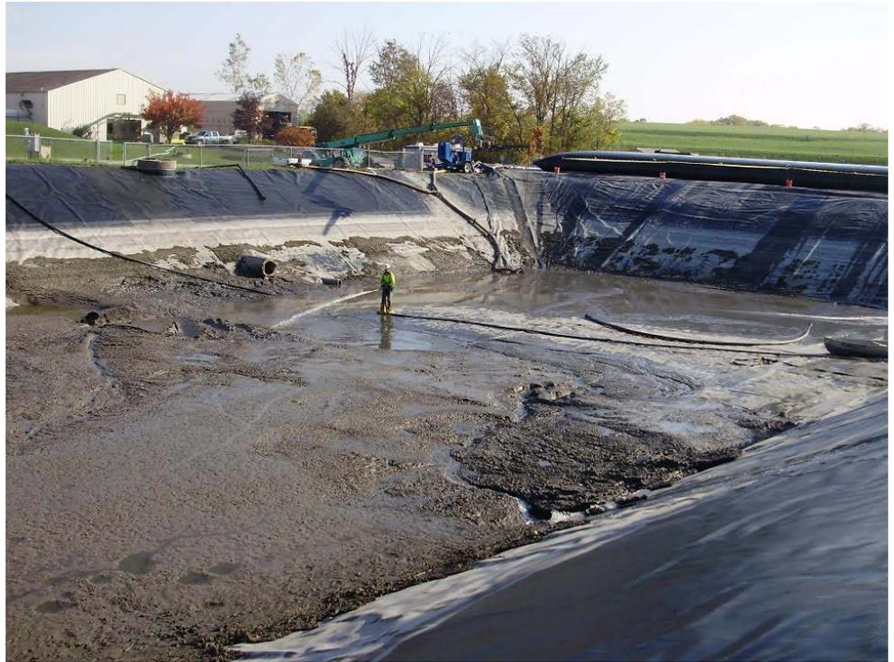
This WaterSolve technician is spraying the solids so they flow to the pump. No harm is done to the liner with process.
