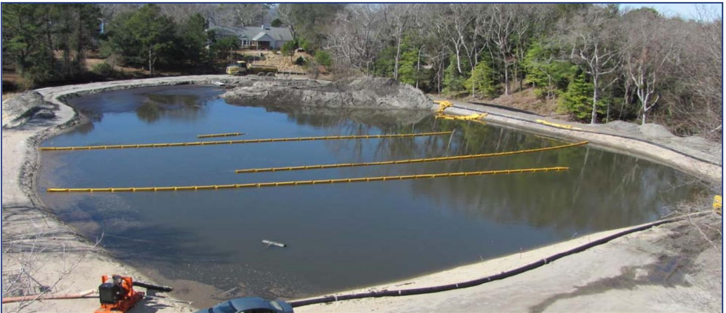
The dredge water is chemically treated before it enters the primary settling lagoon at the top of this photo then makes its way back and forth through the turbidity curtains before it crosses over at the orange pump to the secondary lagoon.
