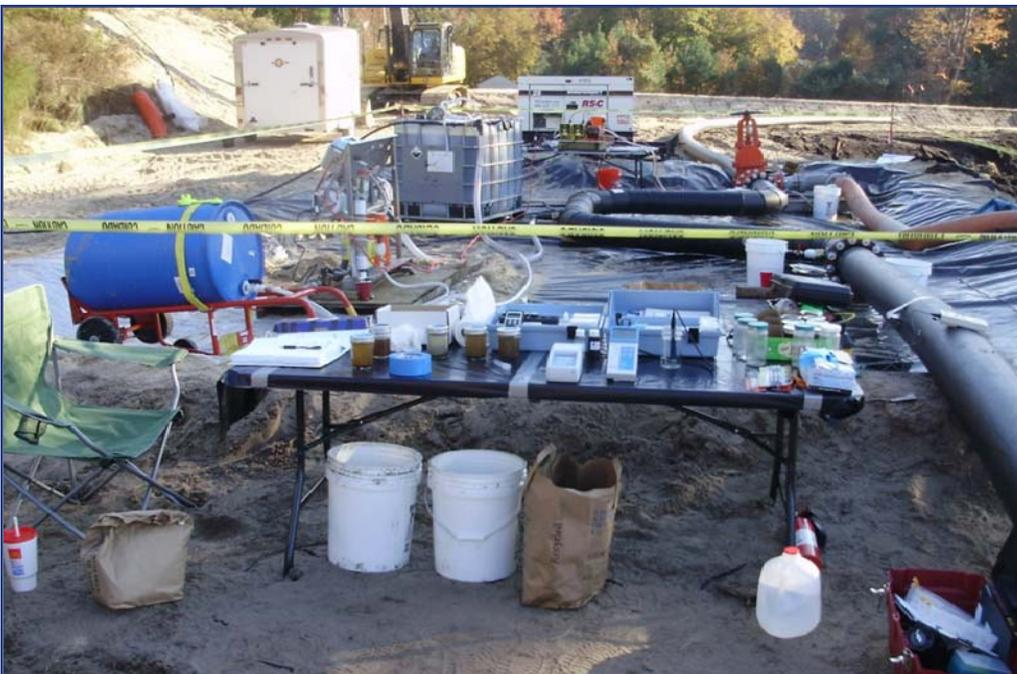
The dual chemical feed system was plumbed to the mixing manifold in the containment area to assure chemical containment of any spills and easy cleanup. The table in front provided a field lab for jar testing and monitoring of the discharge water. This area was later covered with a tent, providing protection from the elements.
