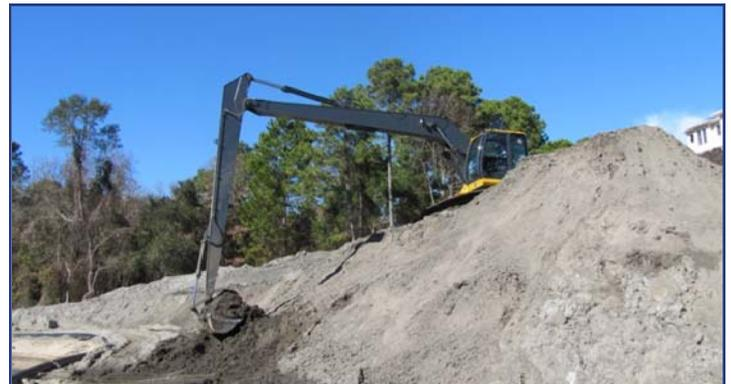
The long reach excavator dipped sand and mud out of the lagoon to maintain settling space for the water. It was then hauled and stockpiled for distribution at the end of the project.
