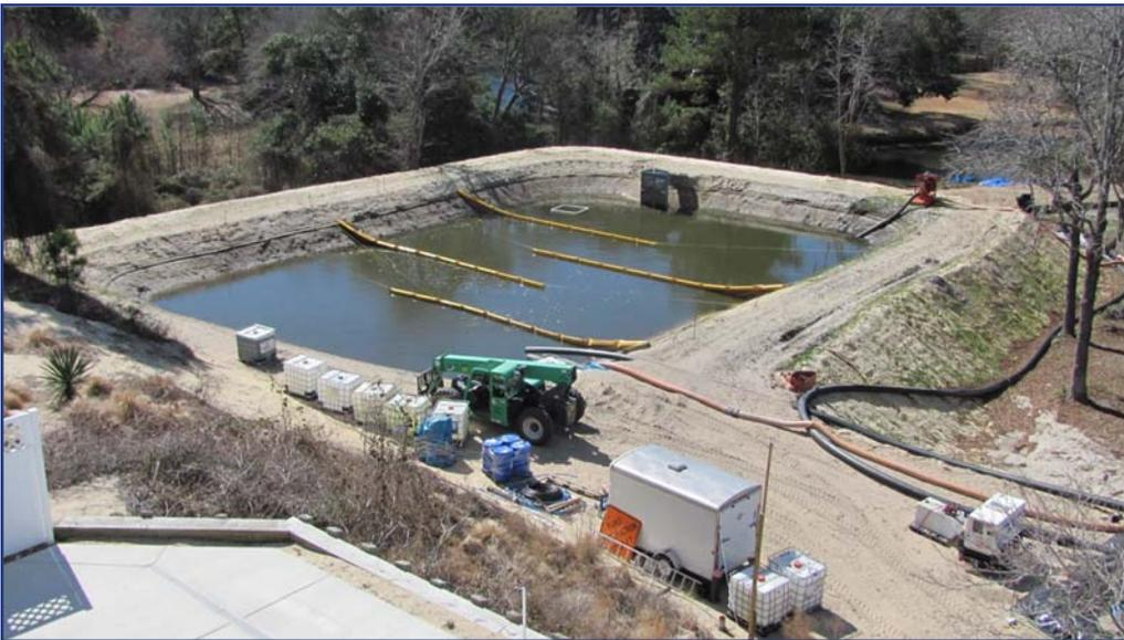
The water crosses over to this secondary lagoon and makes its way to be discharged at the gray flash board riser or the white discharged skimmer. If the water does not meet the requirements, it is circulated and retreated using the orange pump in the upper right of the photo.
