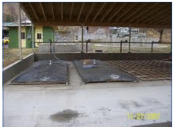
Geotube® units drying area.
