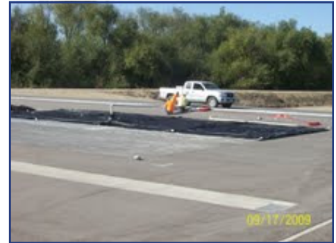
Setting up Geotube® container.
