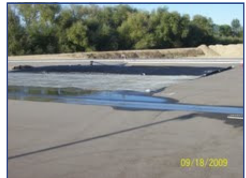
Filling Geotube® container.
