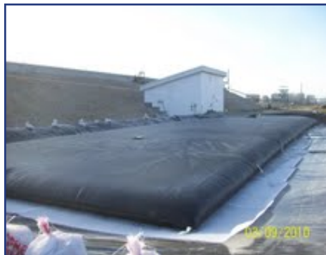
Dewatering of Geotube® container.
