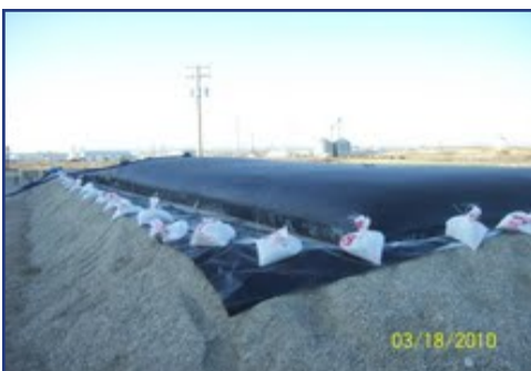
Geotube® container filled and dewatering.
