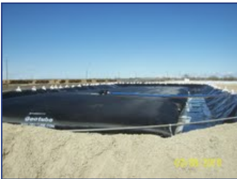
Filling and dewatering of Geotube® container in containment area.
