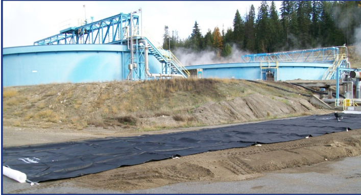
The rolling out of the Geotube® container prior to filling.
