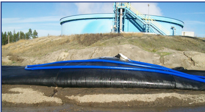
The Geotube® container being filled.
