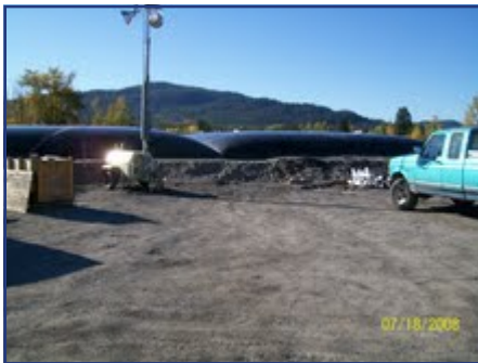
Containment area with Geotube® containers filled .
