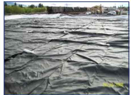
Containment area preparation.
