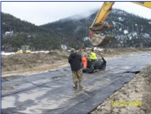
Geotube® unit laid out on scour apron ready to start filling.
