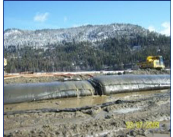
Filling Geotube® units using flatend technology.
