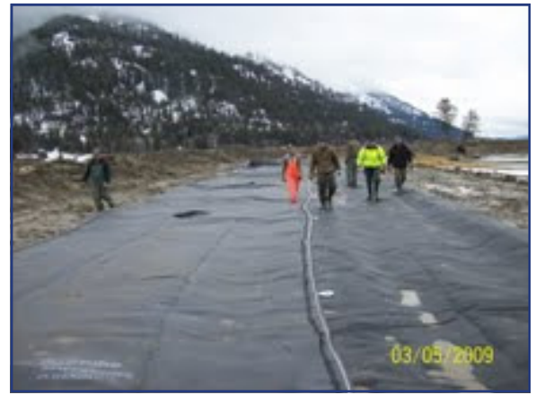
Geotube® unit laid out on scour apron ready to start filling.
