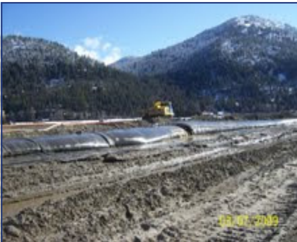
Filling Geotube® units using flatend technology.
