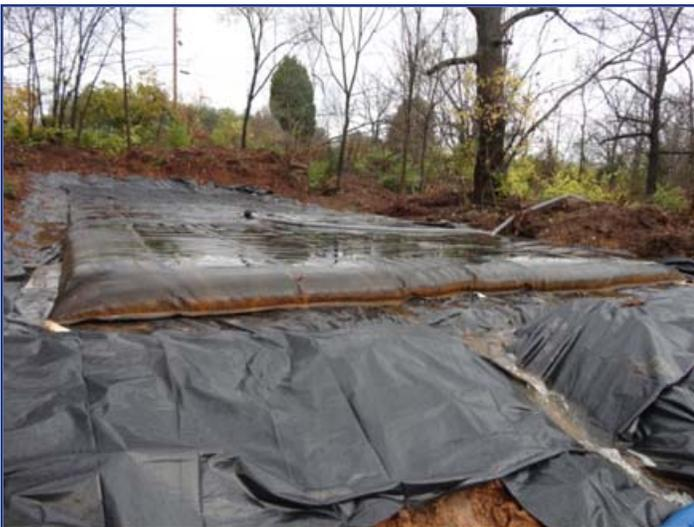
The Geotube container is beginning to fill and the filtrate water is exiting the containment pad and is on its way back to the pond.
