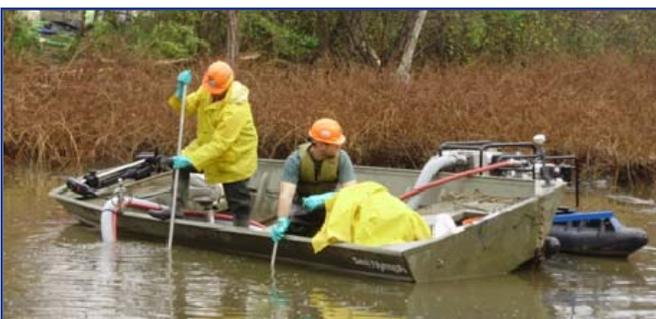
The workers in the boat are pushing the dredge head into the pond sediment and the pond residuals are pumped to the Geotube® container.
