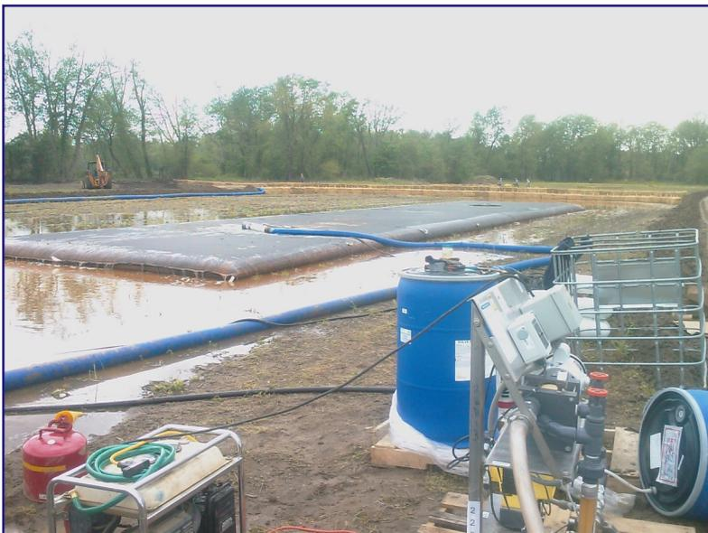
The pipeline residuals are being chemically treated and pumped into the Geotube® container.
