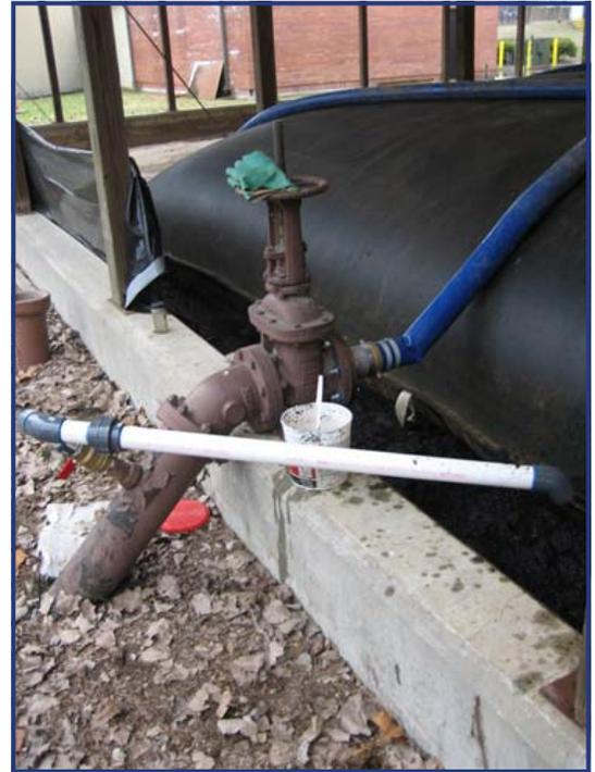
A sampling port was installed just prior to the Geotube® container.
