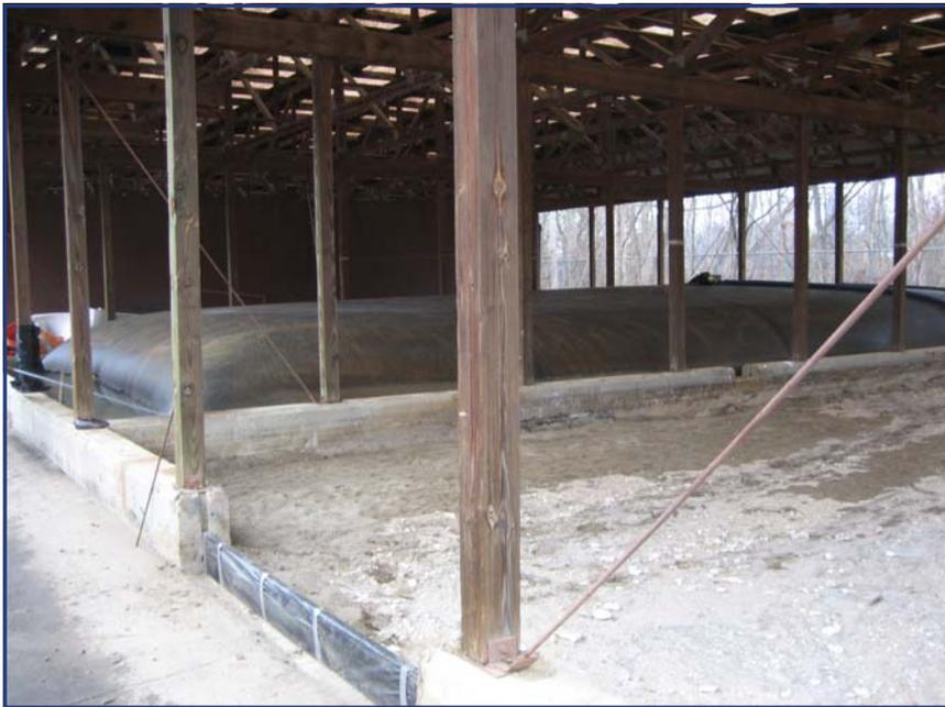
The existing sludge drying beds are in a covered, but open, structure. A Geotube® container was placed in one of the drying beds as shown above.
