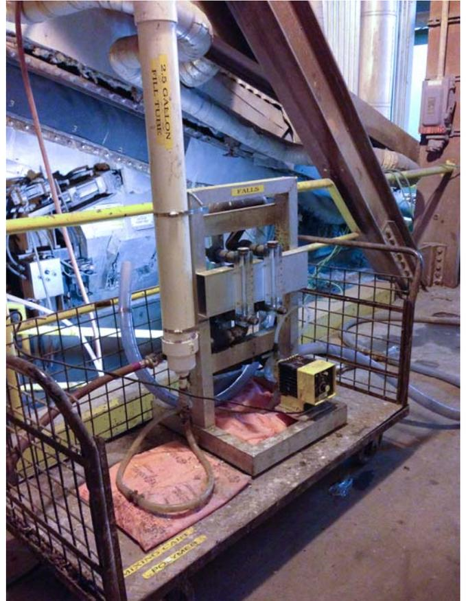
In the picture above the tan tube was designed by the facility personnel and made a effective tool to enhance the polymer make-down unit. Below the polymer injection connection to either unit 1 or unit 2.
