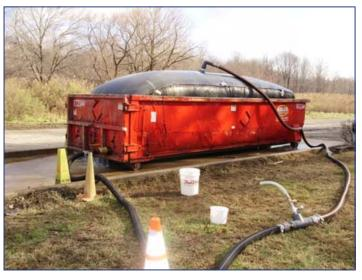
The 20 cubic yard Geotube® is placed in the dewatering dumpster. A sample port in the lower right of the photo provides visual observation for polymer dose adjustments.
