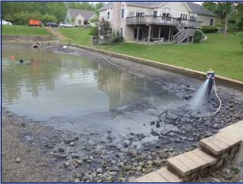
The residual is sprayed to the center of the pond while the divers continue sucking the center.
