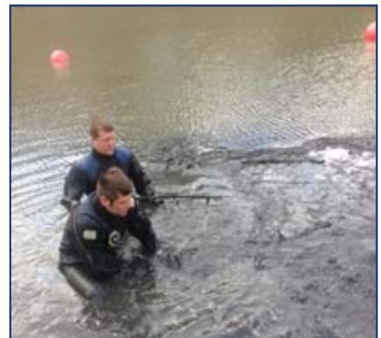
The divers are wearing dry suits while pulling the sediment to the suction hose and removing debris from the pond.
