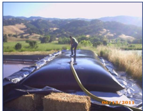
The Geotube® container being filled.
