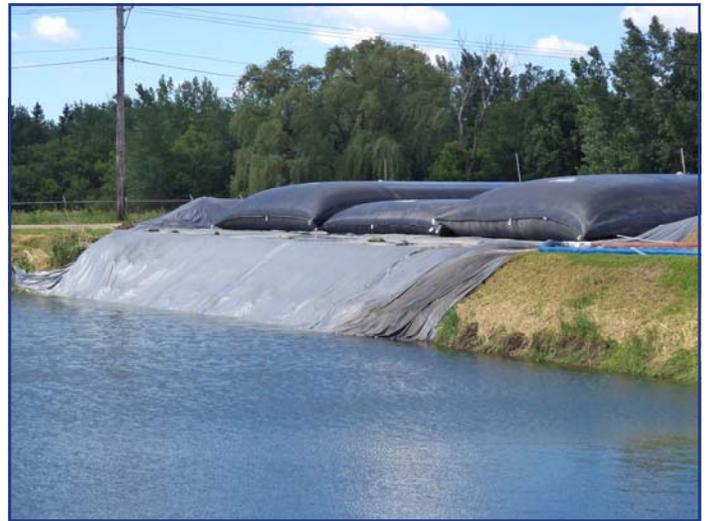
The Geotube ® containers are placed on the containment pad adjacent to the holding pond where the filtrate is free to enter.
