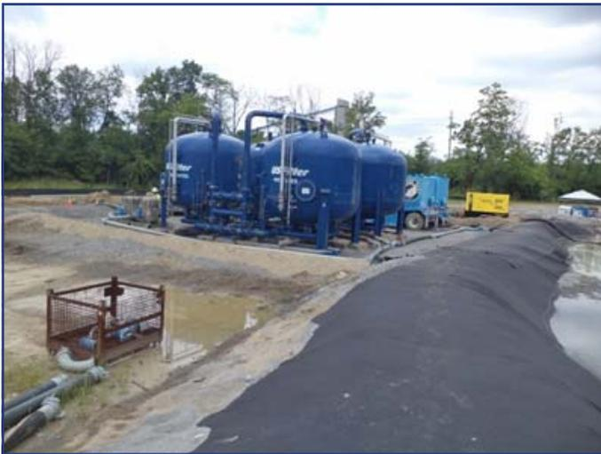
This water treatment plant removed any remaining contaminants from the filtrate water before returning it to the creek.
