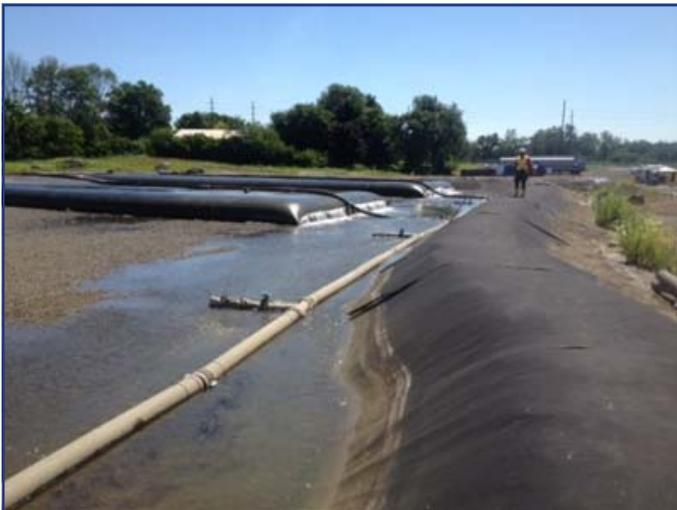
The Geotube® containers are placed in containment pad on a gravel base. The 8” HDP pipeline delivers the residual to the tubes.
