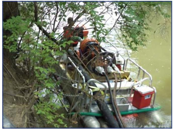
A 6’ hydraulic pump was placed on a raft in the creek. Two 4” hoses were used to suck the residual from the creek into the pump.
