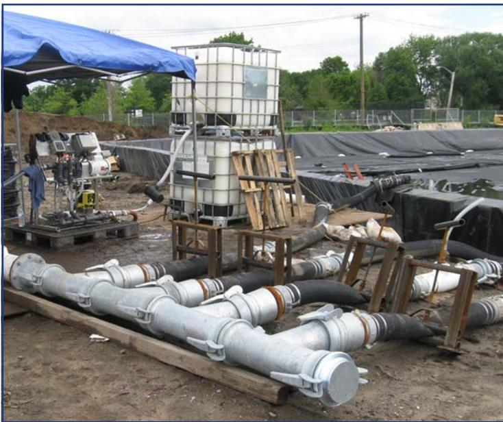
On left feeding polymer into the header system with the 6" pinch valves.
