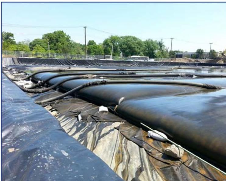
Multiple Geotube® containers dewatering after 3 days of operation.
